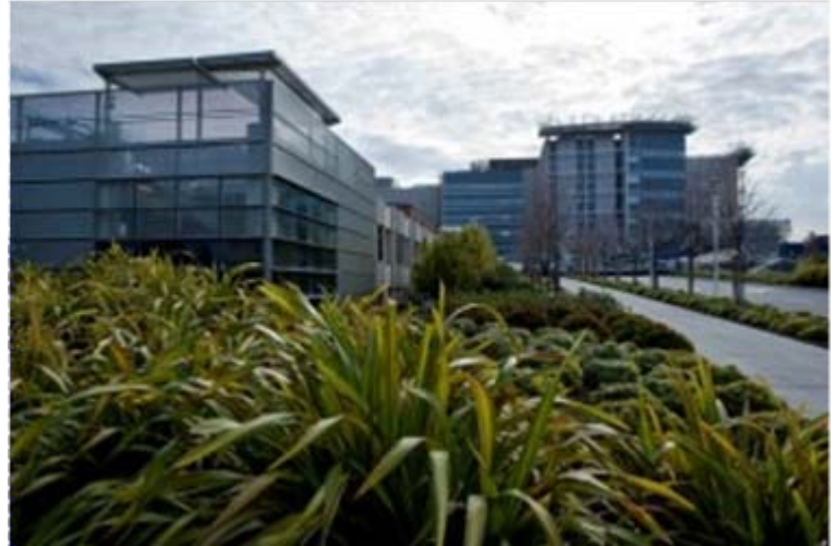
New Mills-Peninsula Medical Center under construction, opening November 2010
